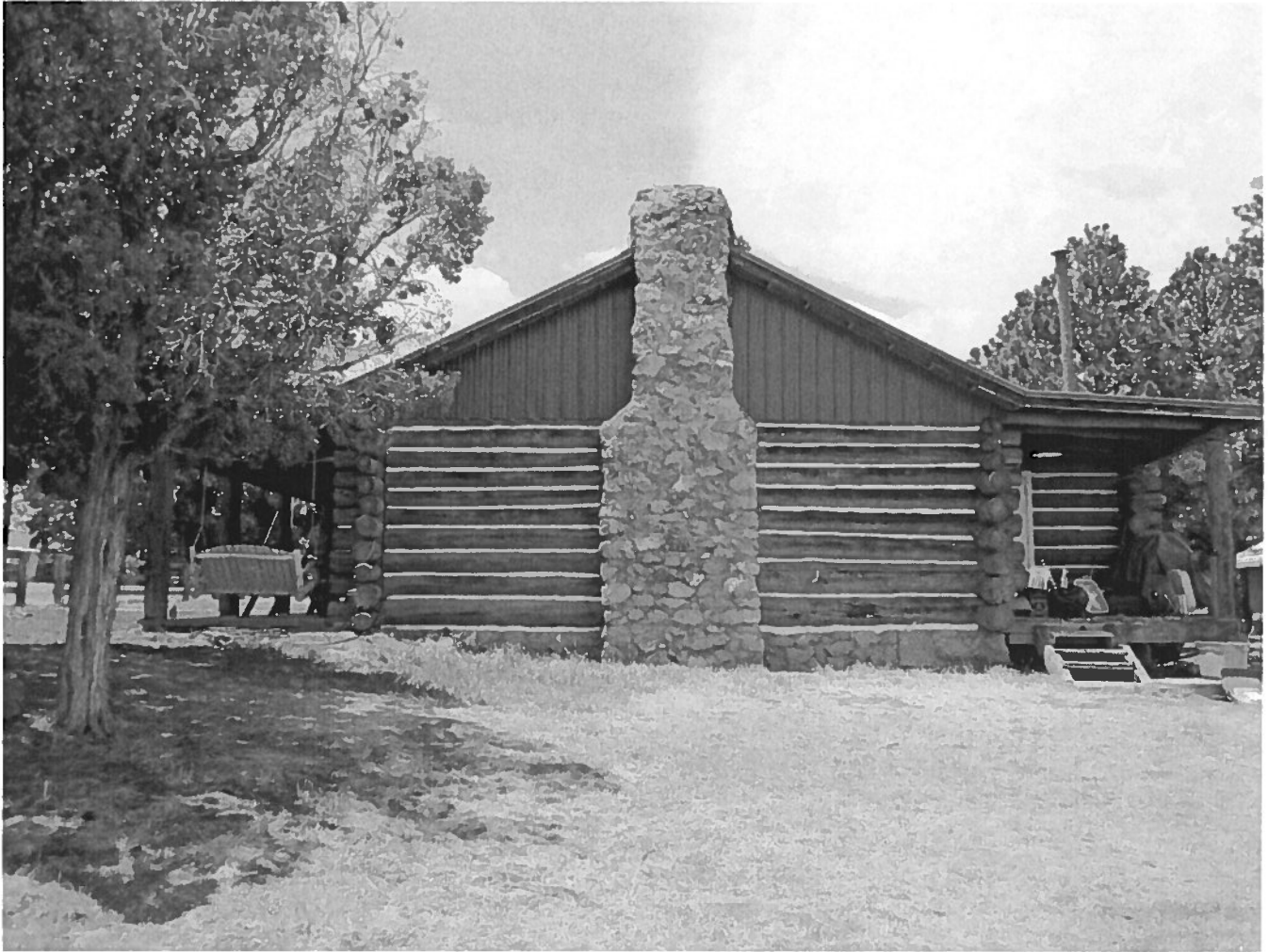
Photograph 2 of 4 East Elevation
